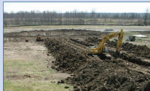
Above: Construction of a levee berm.
